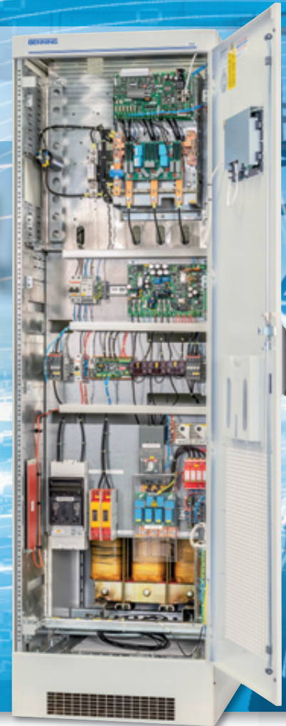
Figure 2: THYROTRONIC Rectifier with interior view
